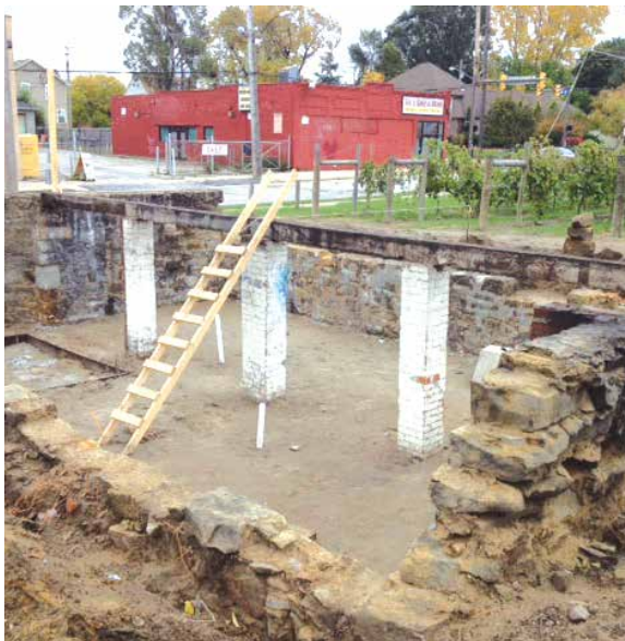
Hough Biocellar under construction in 2013.
